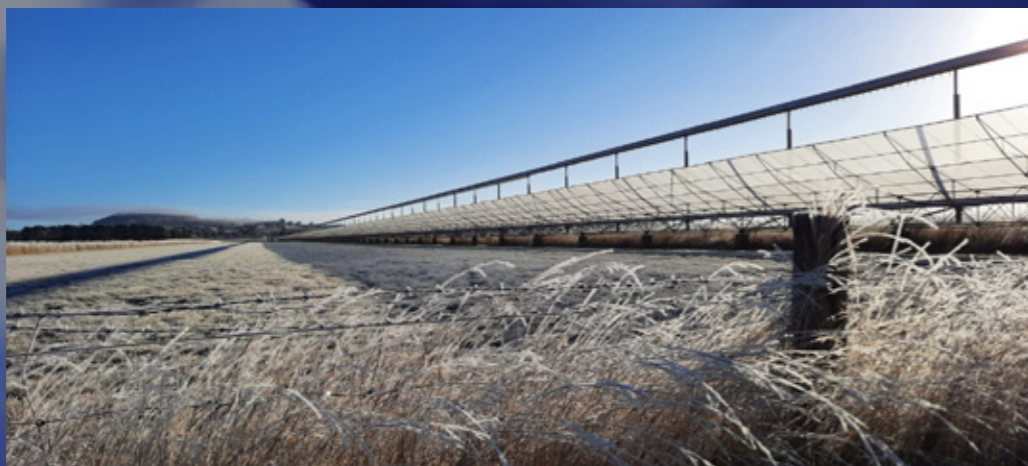
Molonglo Observatory Synthesis Telescope (MOST) is a parabolic cylindrical antenna located near Canberra. Credit: Dr Chris Flynn, OzGrav-Swinburne University of Technology
